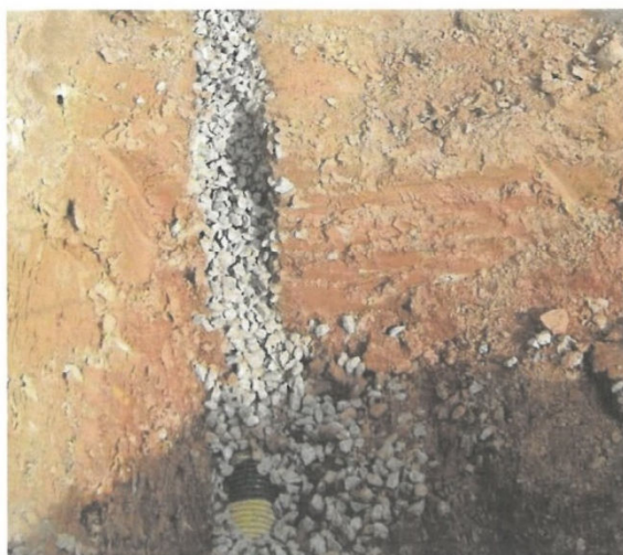
Figure 37. Washed gravel permeable fill over drain
