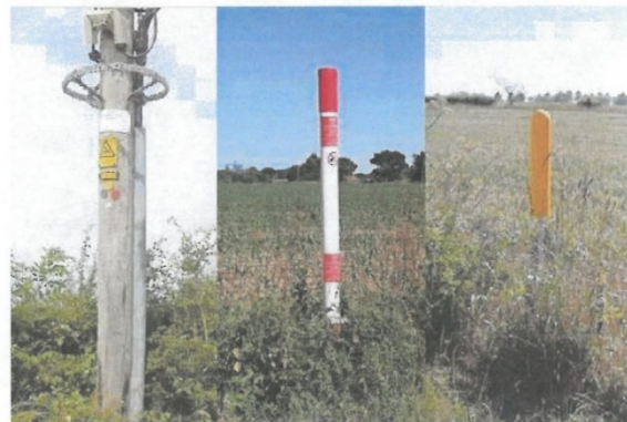
Figure 18. Signs indicating potential underground hazards
