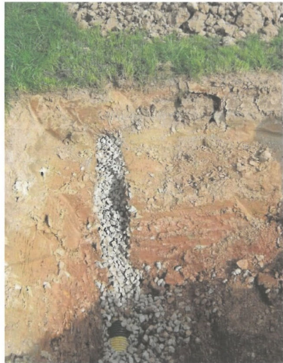
Figure 34. Permeable backfill in trench over drain
