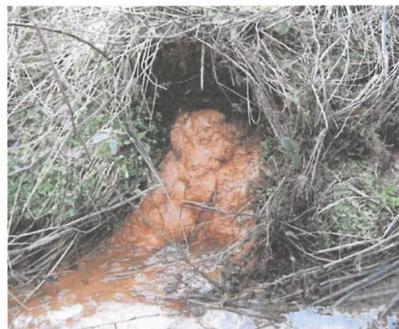
Figure 24. Drainage outfall blocked by ochre
