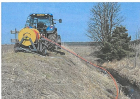
Figure 23. Drain jetting
