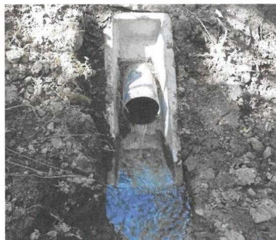
Figure 38. Precast concrete headwall (type K)
