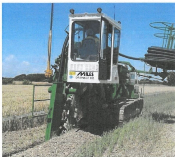
Figure 31. Installing land drains with laser gradient control
