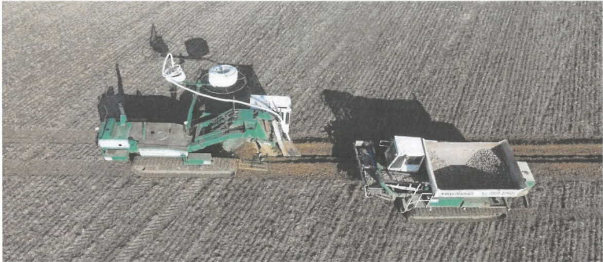
Figure 28. Installing land drains and stone backfill
